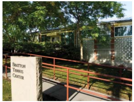
Whitman College, Walla Walla, Washington will install a rooftop solar array this year.
