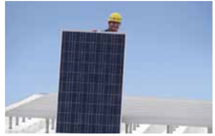
Solar panels are installed at Walla Walla Community College
