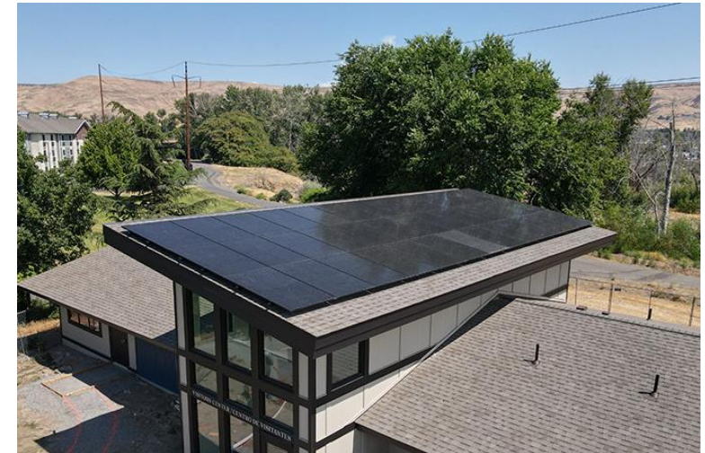
Greenway Foundation Visitor's Center, 15.33 kW solar array
