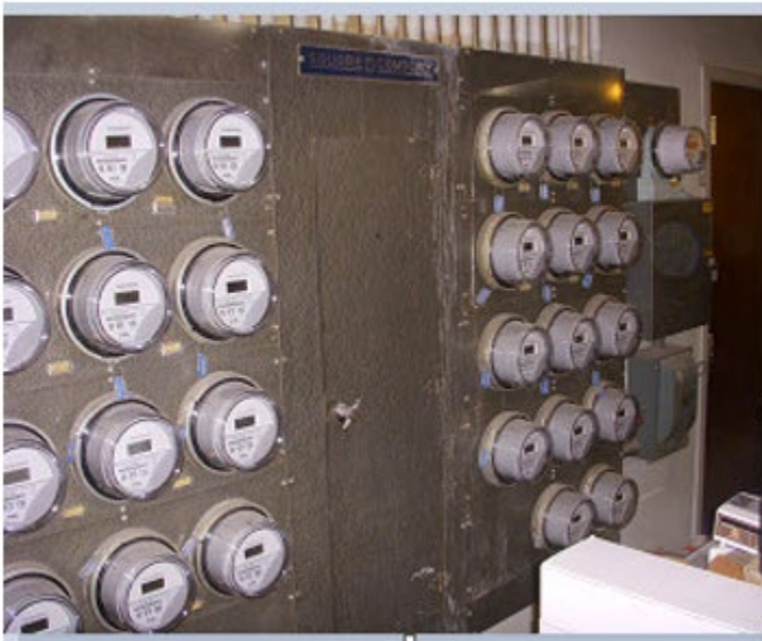
Figure 2. Ganged Meter Sockets
