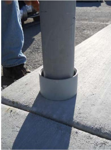
**Figure 23—Installing Conduit through Concrete**
