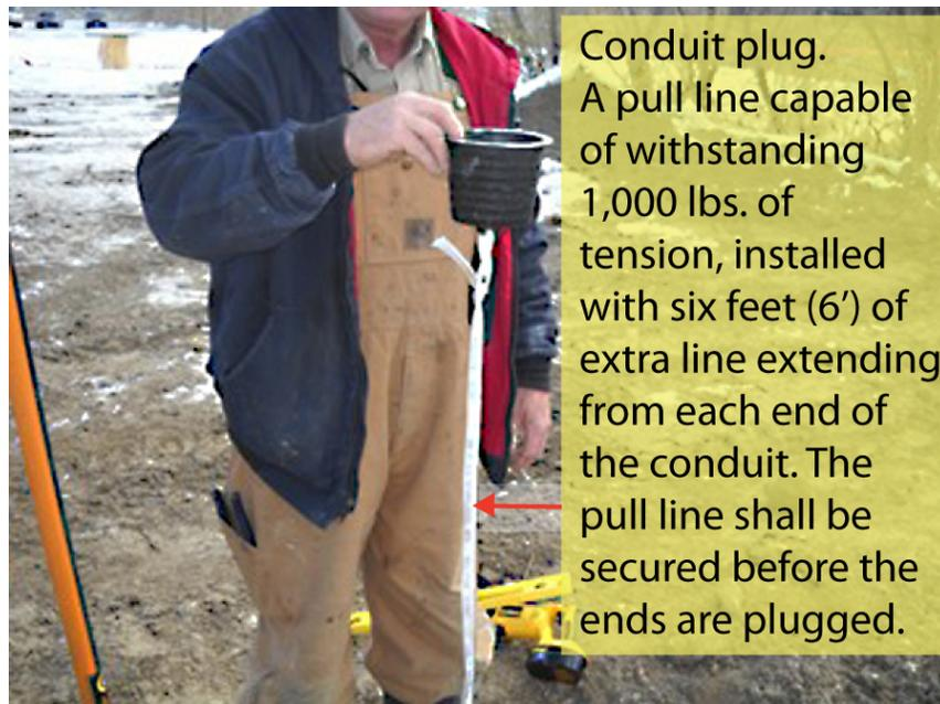
**Figure 26—Conduit Plug and Pull Line**
