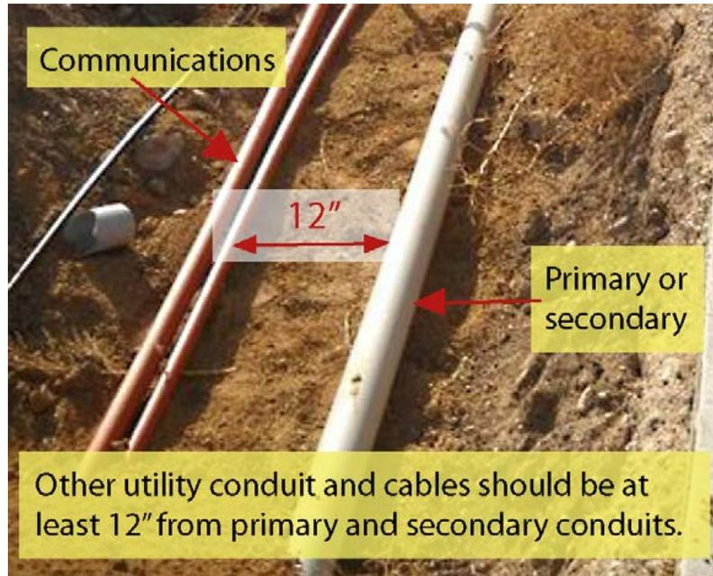
**Figure 10—Joint Trench for Primary/Secondary with Communication**
