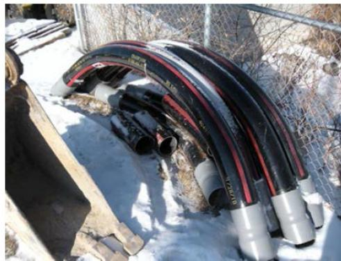
**Figure 15—Fiberglass Sweeps with PVC Ends**
