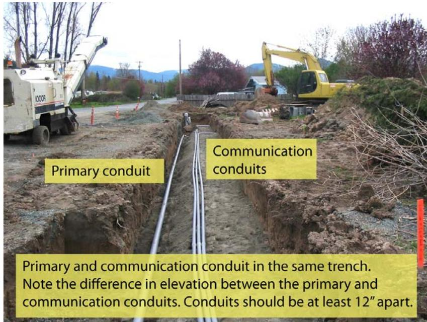
**Figure 8—Power and Communication Conduits in Trench**
