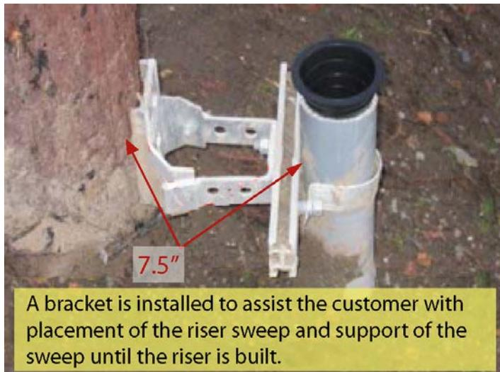
**Figure 30—Riser 7.5" from Pole, Bracket**
