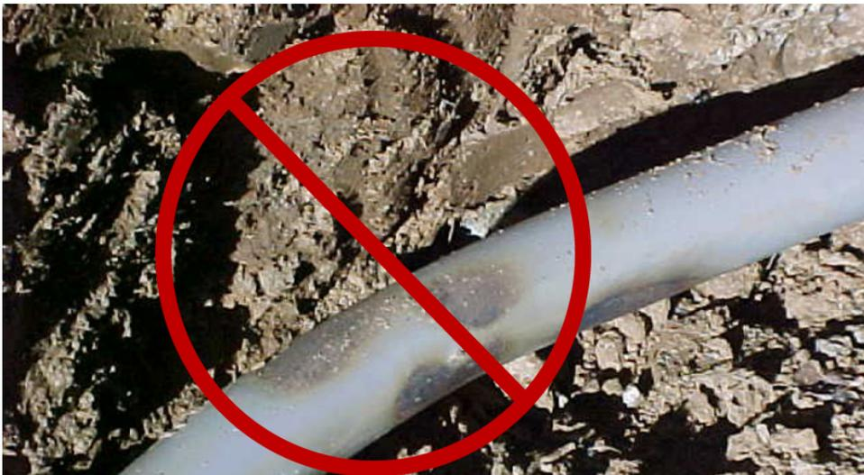
**Figure 17—Field-Altered Sweep – Damaged PVC**
