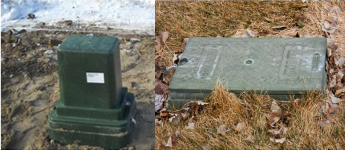
**Figure 58—Above Grade Pedestal and Flat Lid Installed on Secondary Boxes**
