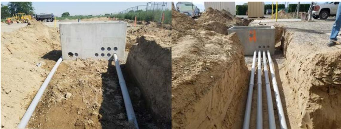
**Figure 20—Typical Conduits Attached to a Padvault and Communication Conduit Next to Padvault**
