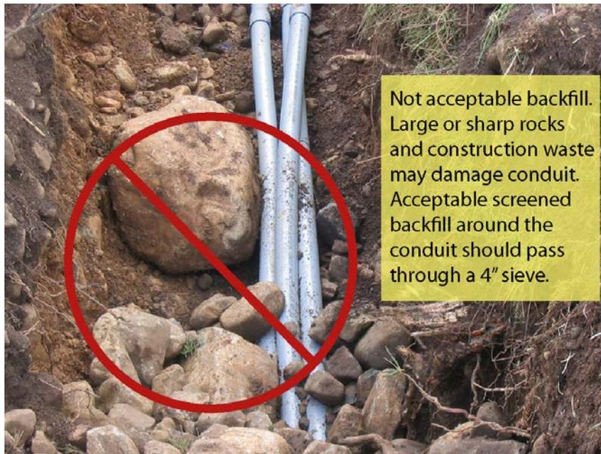
**Figure 13—Unacceptable Backfill**
