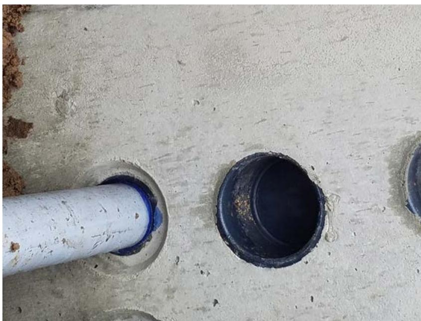
**Figure 22—Proper Installation of Conduit into Term-A-Duct**
