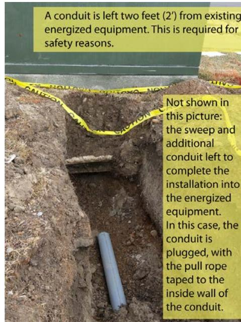
**Figure 19—Installing Conduit to Existing (Energized) Equipment**
