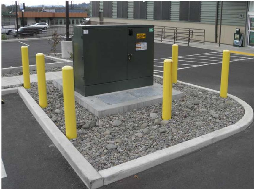
**Figure 46—Barrier Posts, Example**
