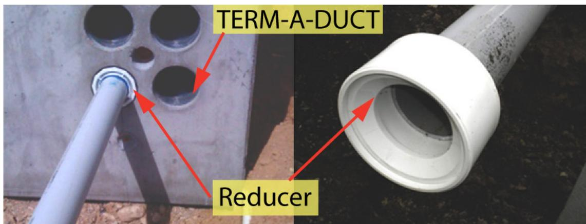
**Figure 21—Reducer Used for Conduit Entering the Padvault**
