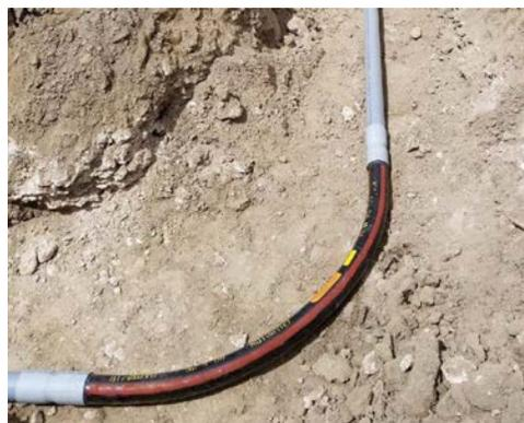
**Figure 16—Field-Installed Elbow**
