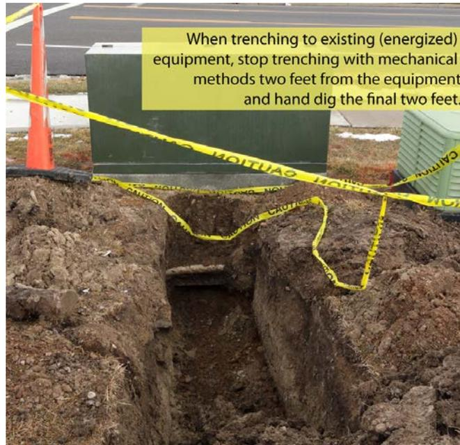
**Figure 3—Trench to Energized Equipment**
