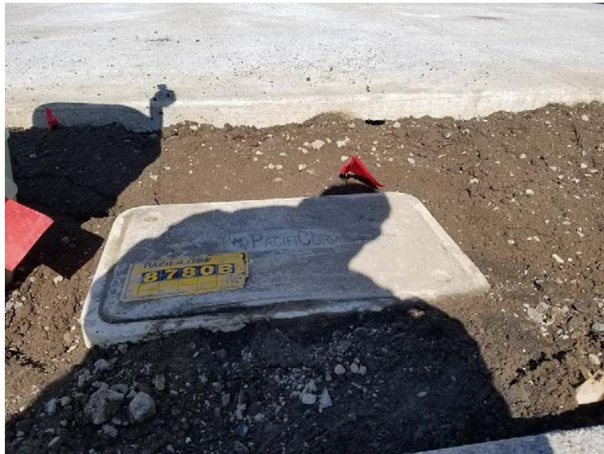
**Figure 61—Installed Fibercrete Secondary Box Base and Flat Lid**
