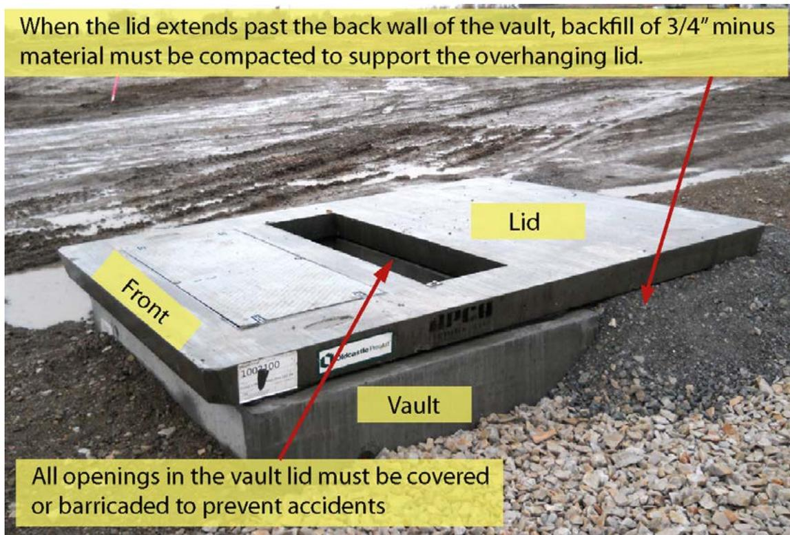
Figure 47—Correctly Installed Padvault in Non-Pedestrian Area
