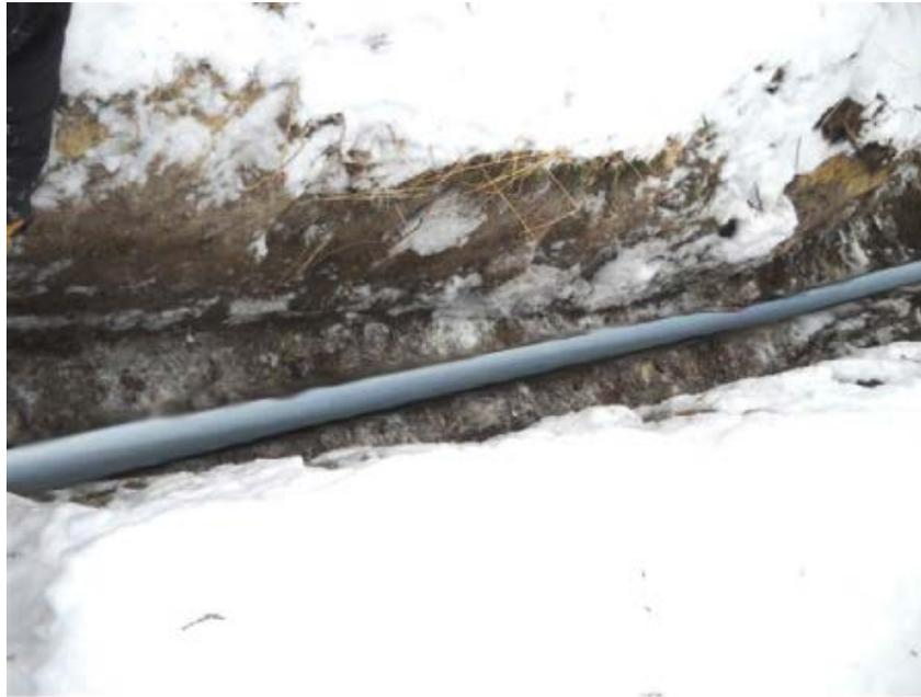
Figure 5—Typical Conduit Trench
