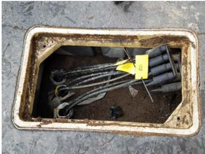
**Figure 65—Example of Proper Conduit Installation for Flat Lid Top**
