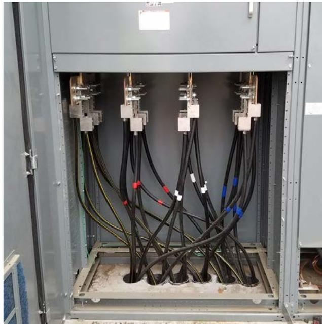
**Figure 40—Example of Correct Conduit Installation**
