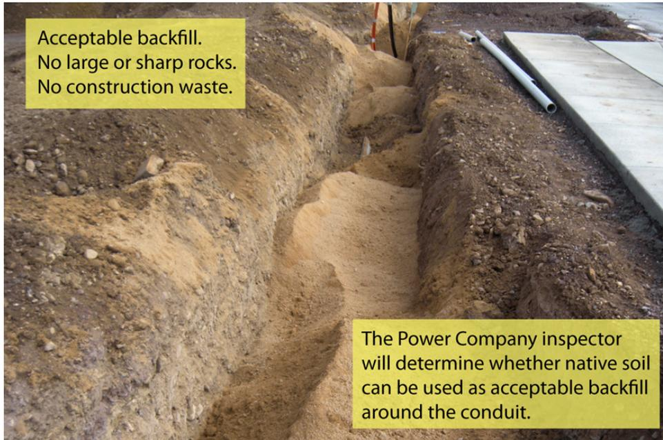
**Figure 12—Acceptable Backfill**
