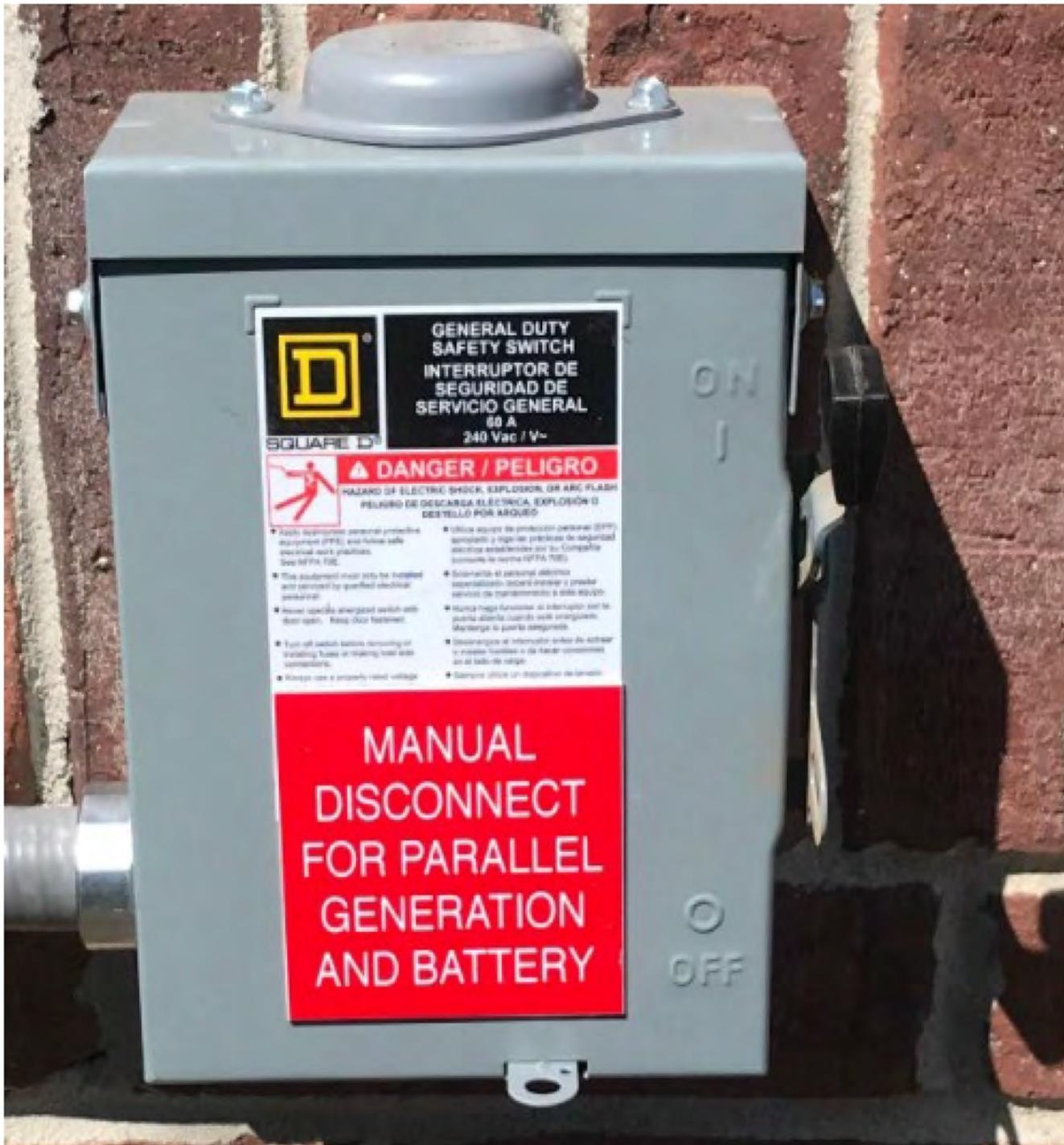
This is an example of using an E-stop button (or other switch) that can shut off the battery system.
